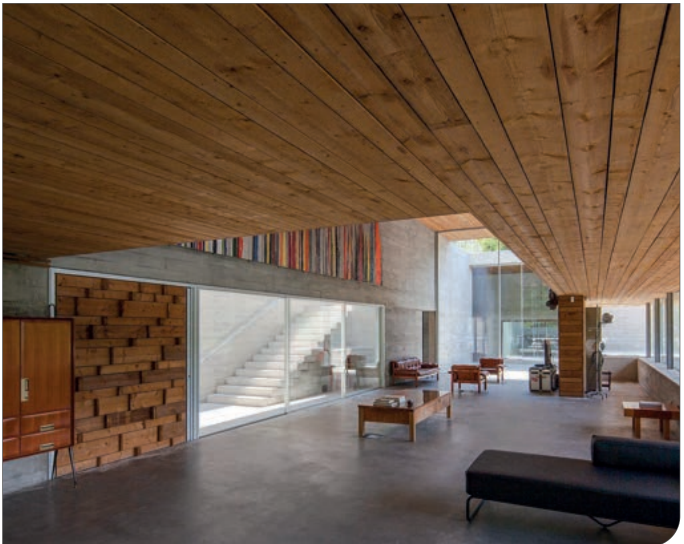
Figure 38. ThermoWood® ceiling in Portugal
