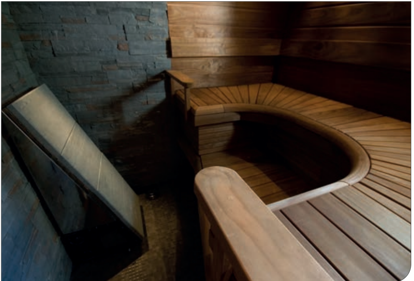
Figure 44. Sauna structures made of ThermoWood® products.
