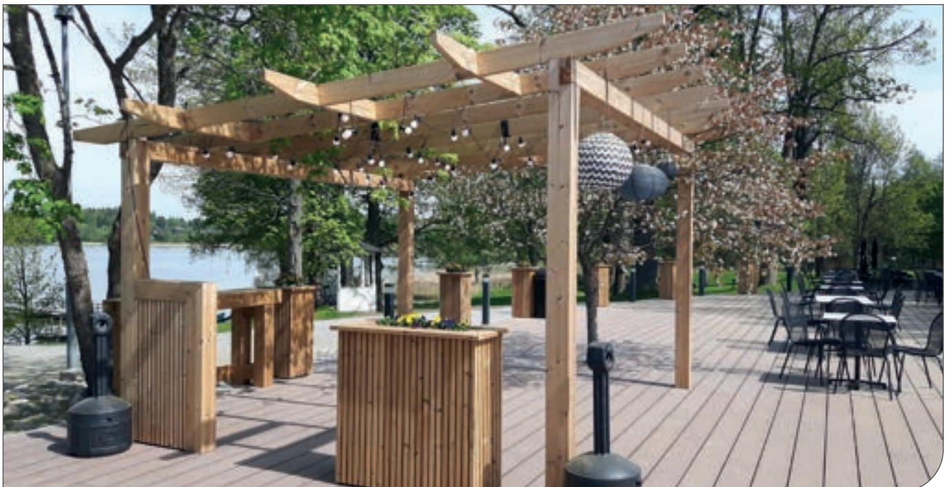
Figure 33. ThermoWood® glue beams in pergola structure
