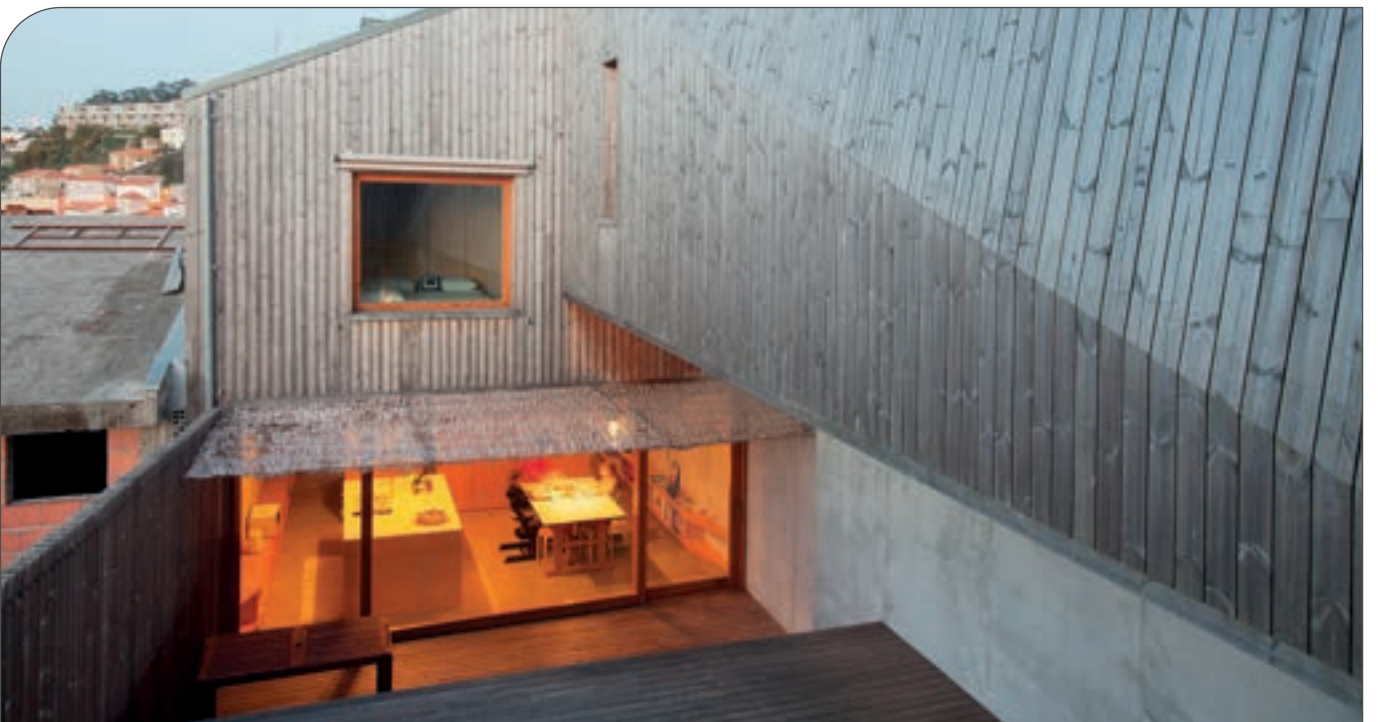
Figure 61. ThermoWood® exterior wall cladding with a naturally weathered appearance in Portugal.
