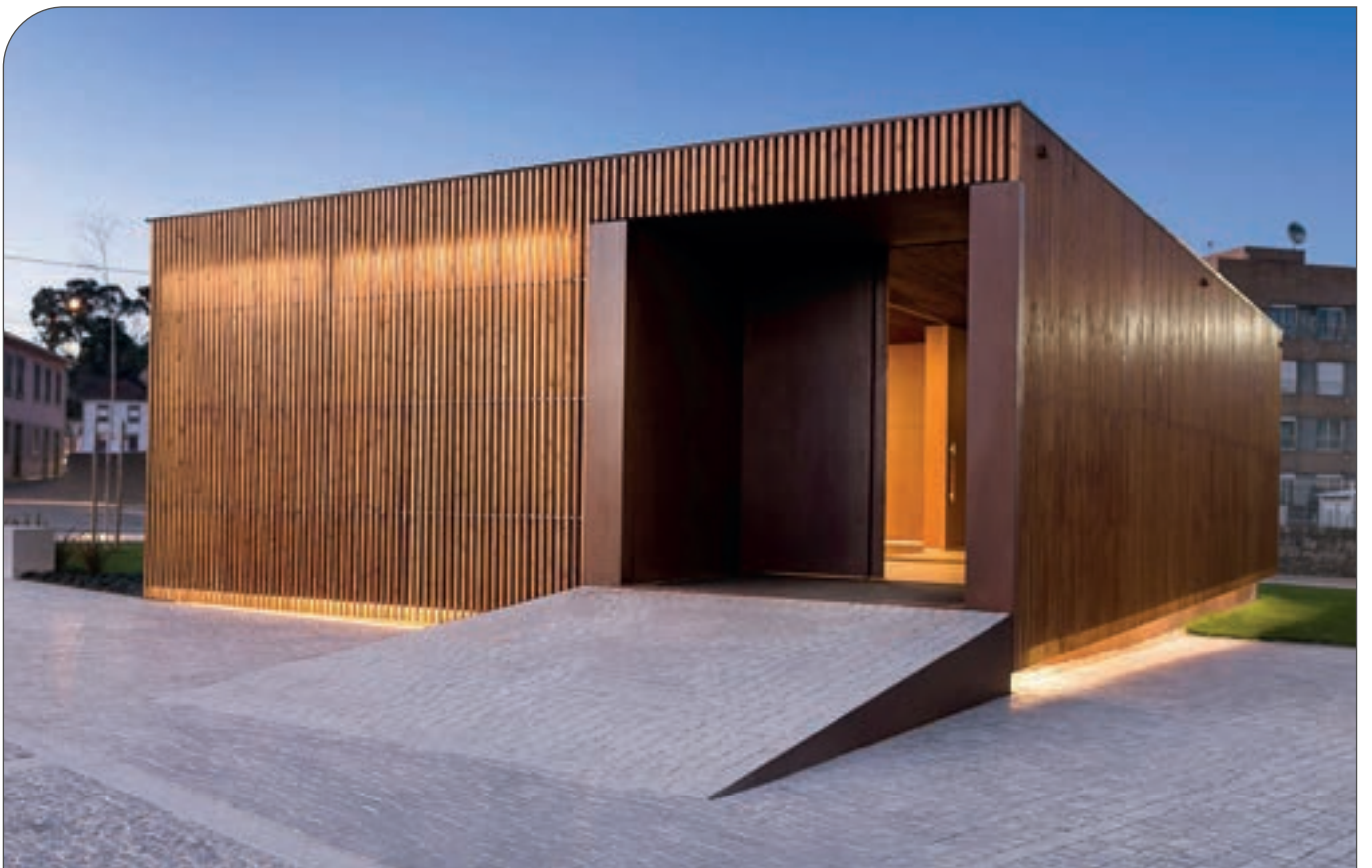
Figure 67. ThermoWood® exterior wall cladding on a Portuguese church.
